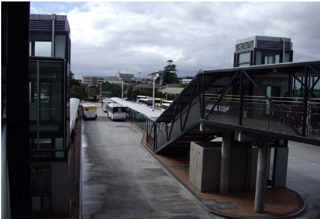
Photograph B4 - Looking towards Moore Street entry to Liverpool Station bus interchange, July 2011.
