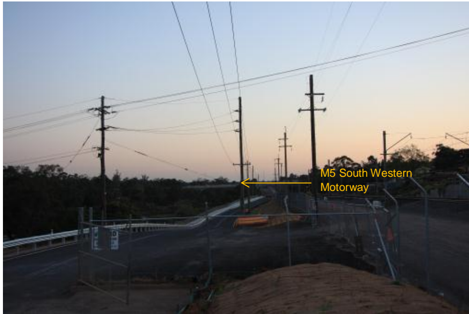
Figure 3 Location L1 view towards Moorebank IMT site which will be the other side of the M5 Motorway
