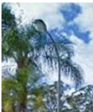
Figure 18A – Goodenough Street cul-de-sac, glass bowl B22 Sylvania luminaire with mercury vapour light source
