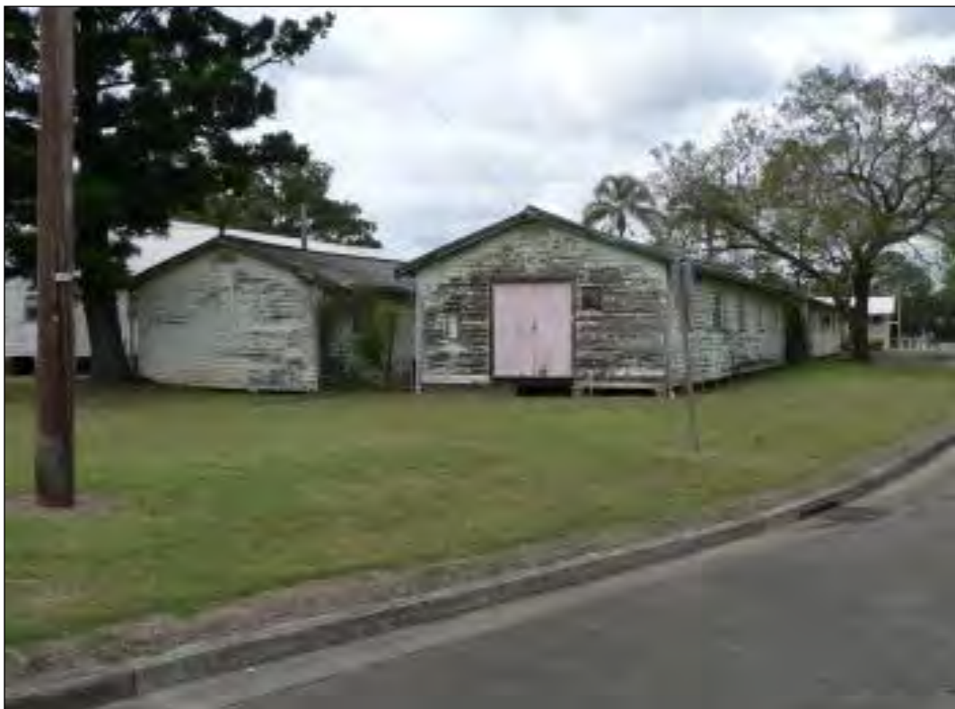
Figure 5.7 Building B36-B39, from the north
