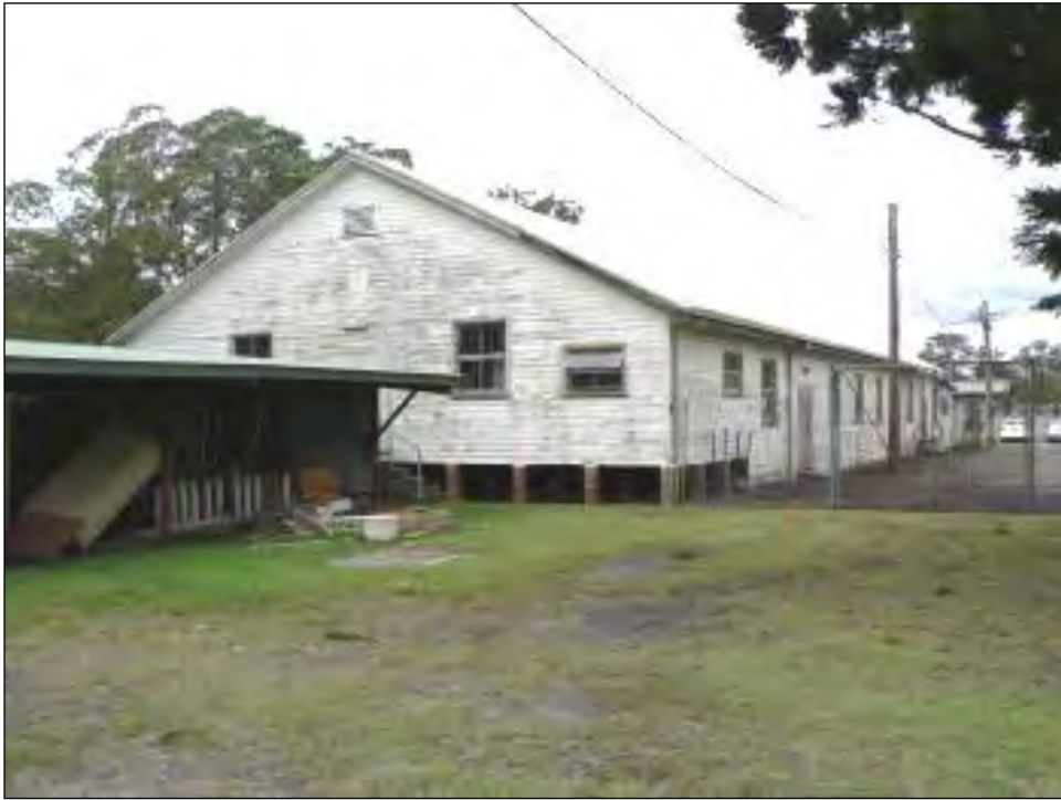
Figure 5.12 Drill Hall Building B40 from northwest
