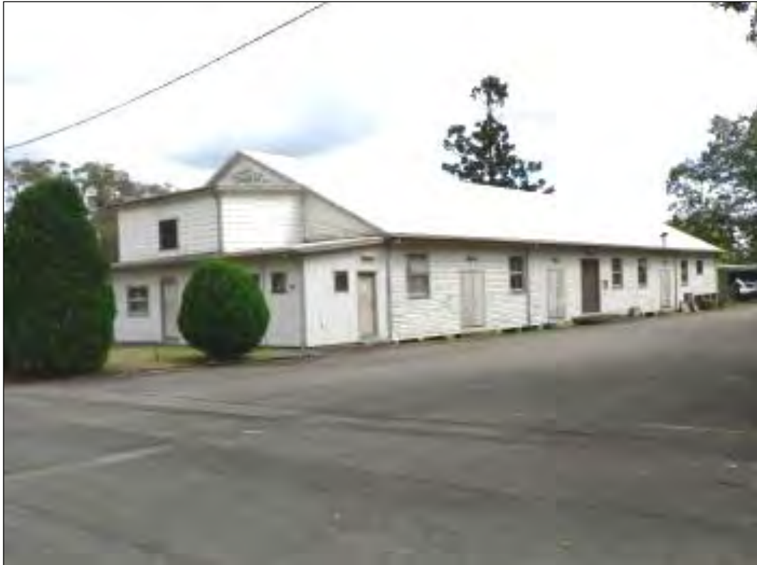
Figure 5.11 Drill Hall Building B40 from southeast
