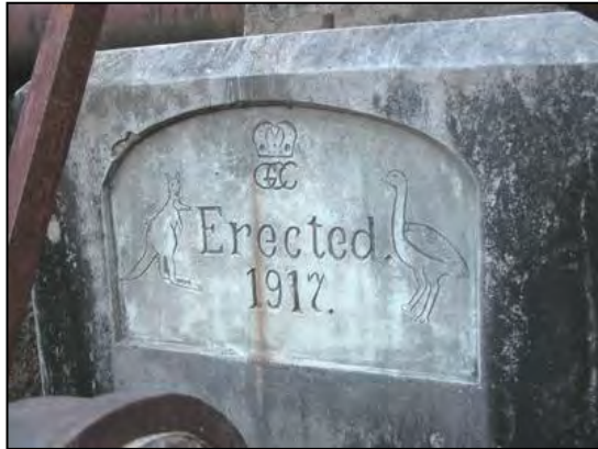
Figure 4.12 Inscription on pier of bridge over Harris Creek (NSW Heritage Office)
