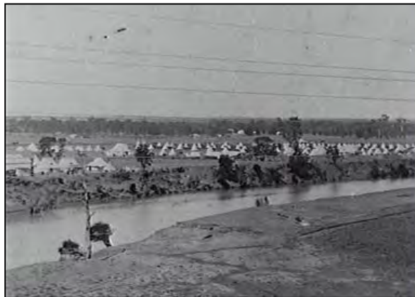
Figure 4.5 View looking east from the railway line across the George's River to Liverpool military camp, 1910-11 (Follan Collection, Campbelltown City Library)
