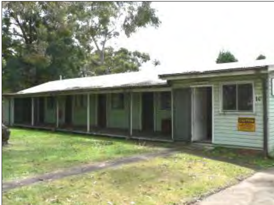
Figure 5.9 Building B47 from southwest
