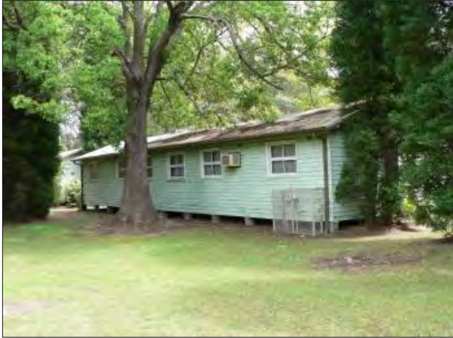
Figure 5.8 Building B44 from southeast
