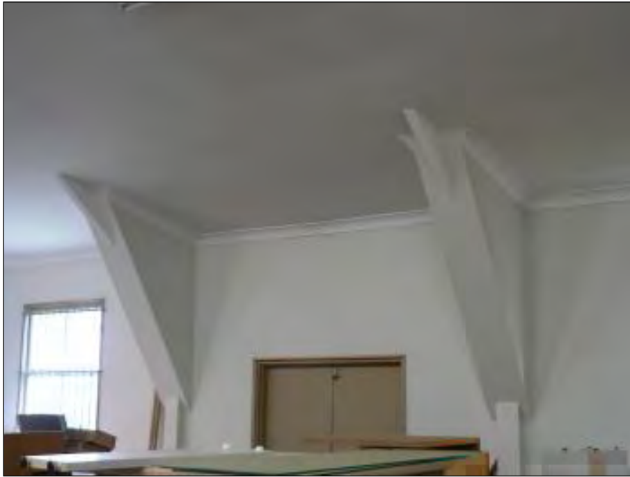
Figure 5.14 Detail of box bracing and altered doorway - Building B40
