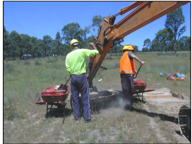
Figure 20 Selection and transporting of excavated deposit
