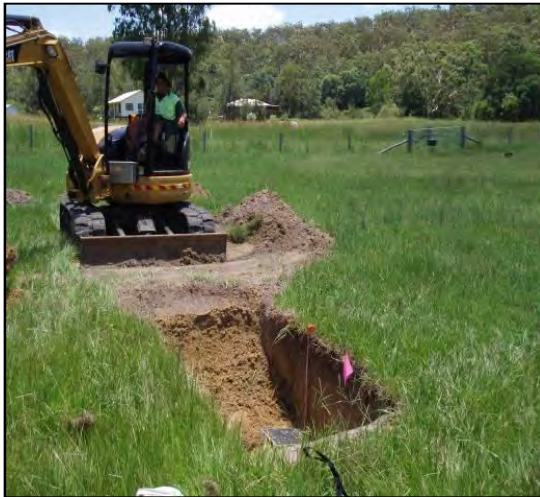
Figure 19 Example of excavation conducted by an excavator
