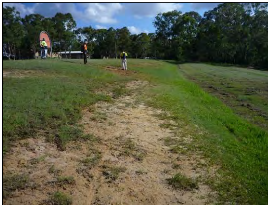
Figure 13 MA5 looking south along edge of terrace
