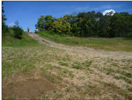
Figure 10 MA4 looking east, note elevated terrace and modified embankment.
