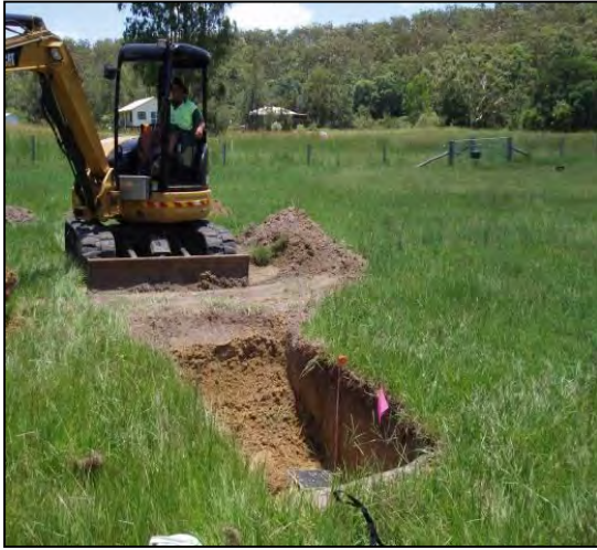
Figure 19 Example of excavation conducted by an excavator
