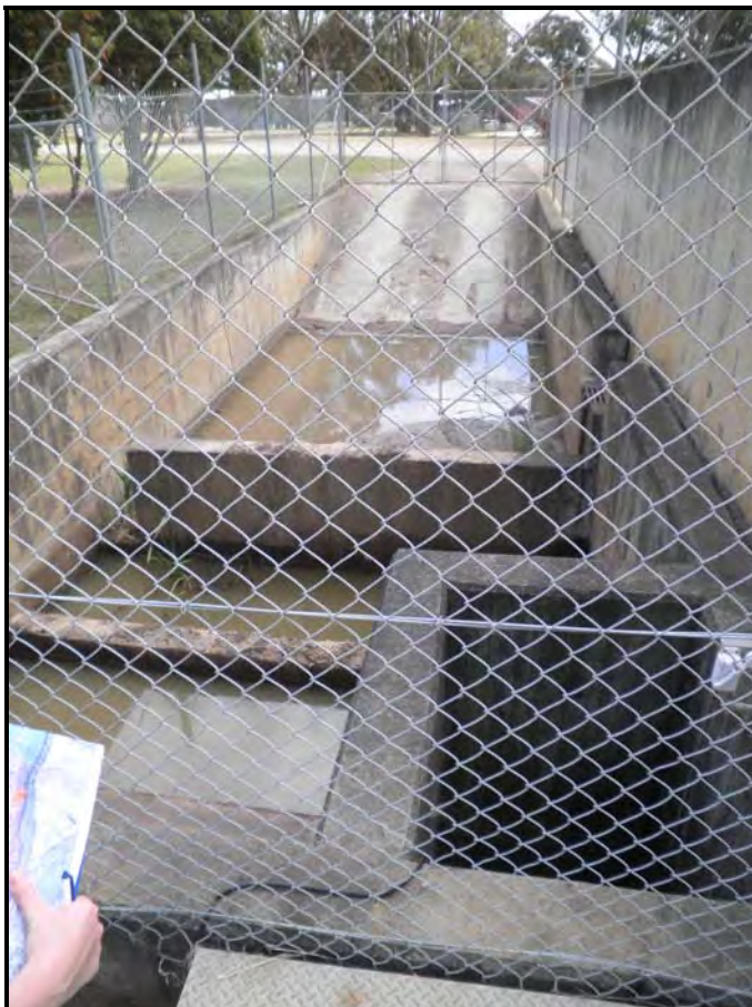
Photograph 46: Oil/water separator pit, PRA Yard.
