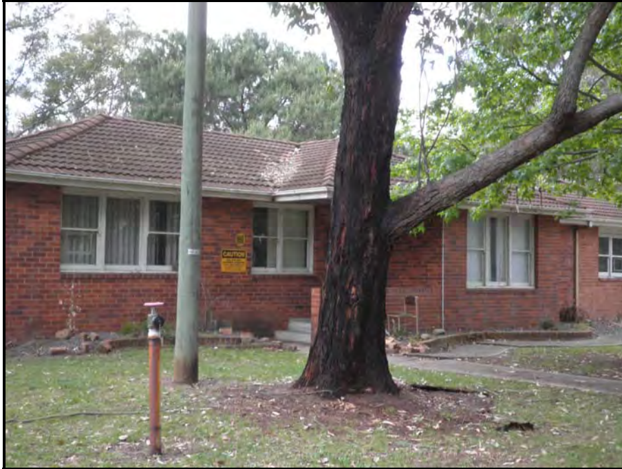
Photograph 13: Building in Jacquinet Court area which is known to contain asbestos. The structure is currently used for training exercises.
