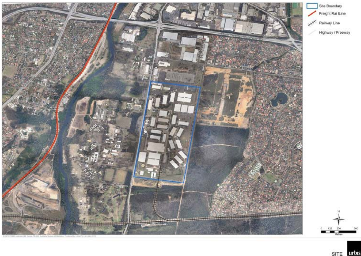
FIGURE 4 – AERIAL PHOTOGRAPH (URBIS 2010)
